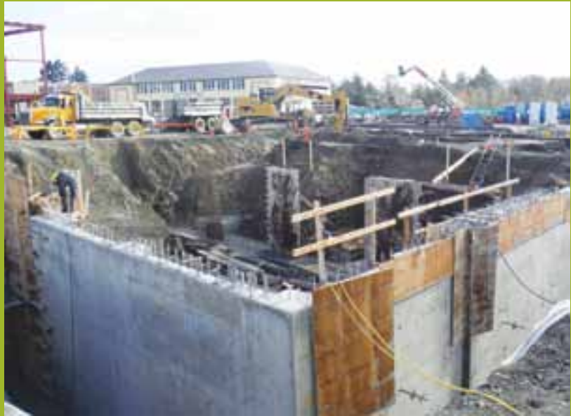
Oak Bay High School basement mechanical room foundation.
