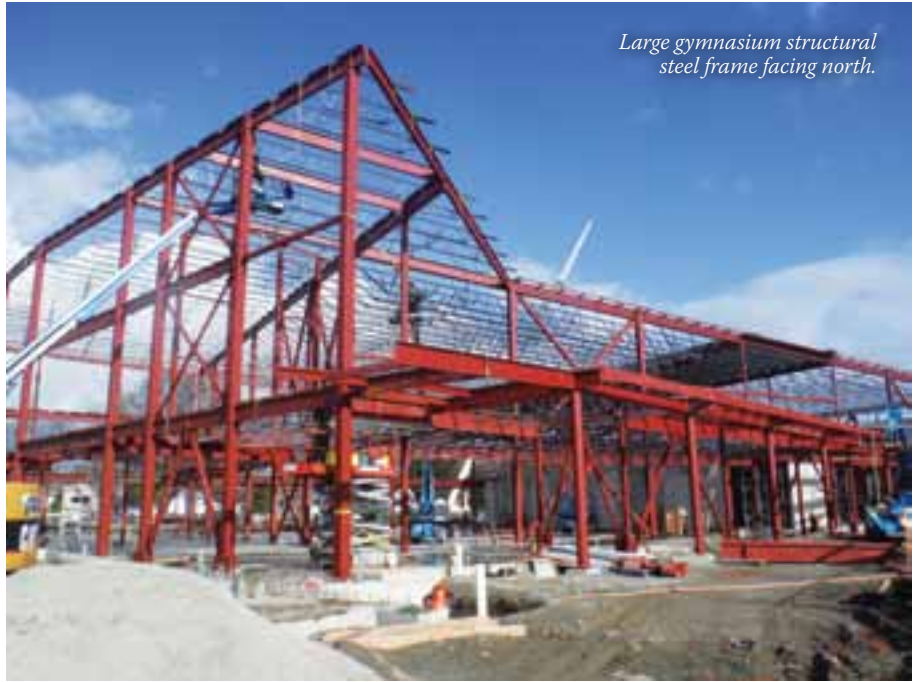
Oak Bay High School replacement project. Foundation and grade slab, structural steel frame.
