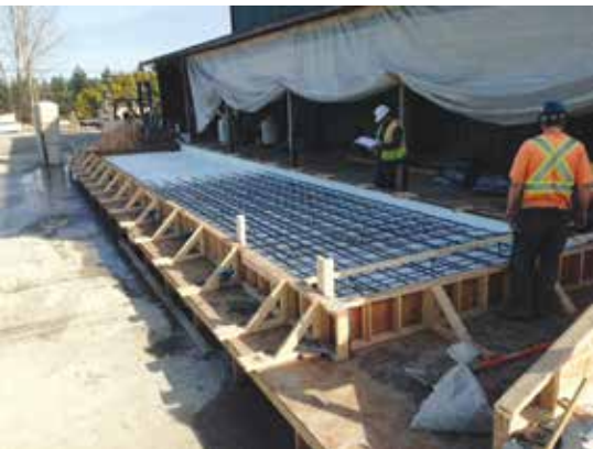
Panel on the steel deck with layer of concrete poured, foam and rebar before second concrete pour.
