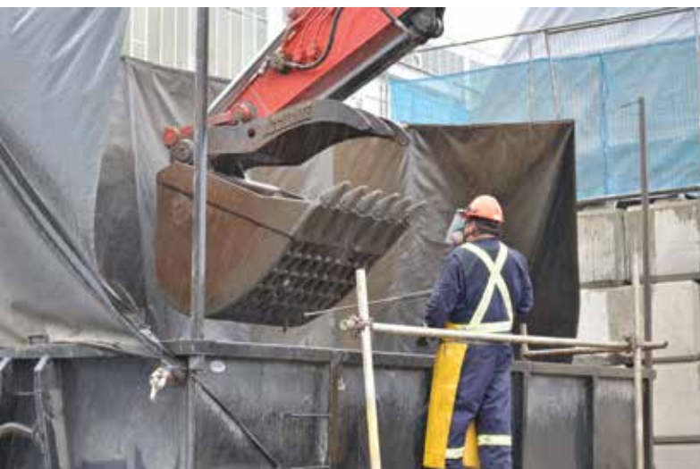
Allterra cleaned and decontaminated every particle of waste on the FMF Cape Breton site to prevent further contamination outside of the project site.
