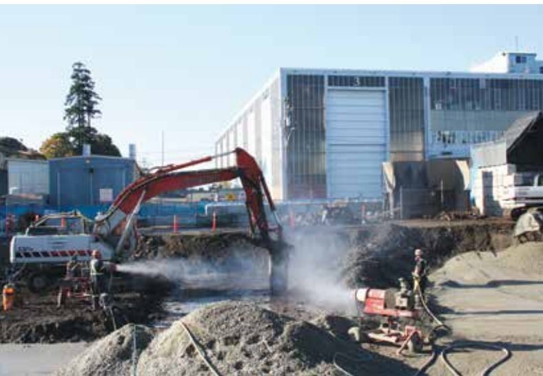
Allterra crews use a water cannon to contain environmental particulates during the injection process.
