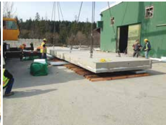
Lifting the panel off the steel deck onto a leveled foam bed on top of 4"x4".
