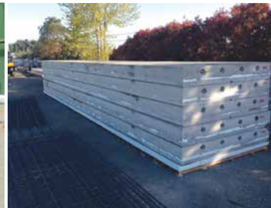
Inventoried panels on a foam bed stalked for shipping to site.
